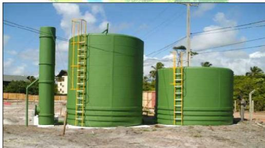
Figura 70 – Reator UASB
